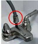
In some RV's the shower is connected with the faucet of the wash basin. The connecting piece between hose and faucet has a plastic nozzle (left picture). Pull this nozzle up so that the water is diverted to the shower head. All showers heads have a slider (right picture). It stops the water flow temporarily to help save water while having a shower.
